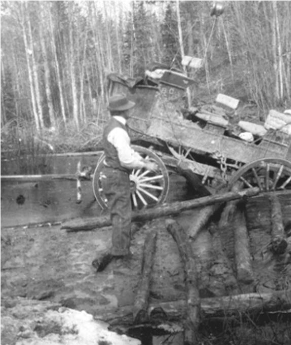
A wagon has slipped off the corduroy road. It is stuck in the mud.
