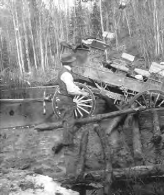
A wagon has slipped off the corduroy road. It is stuck in the mud.
