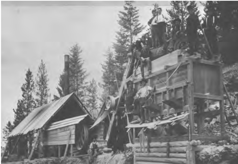
The type of rock crusher used during the building of highways in the Okanagan.
