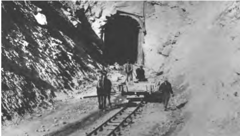
Labourers and a horse-drawn cart at Adra Tunnel near Naramata Photo courtesy of Kelowna Museum
